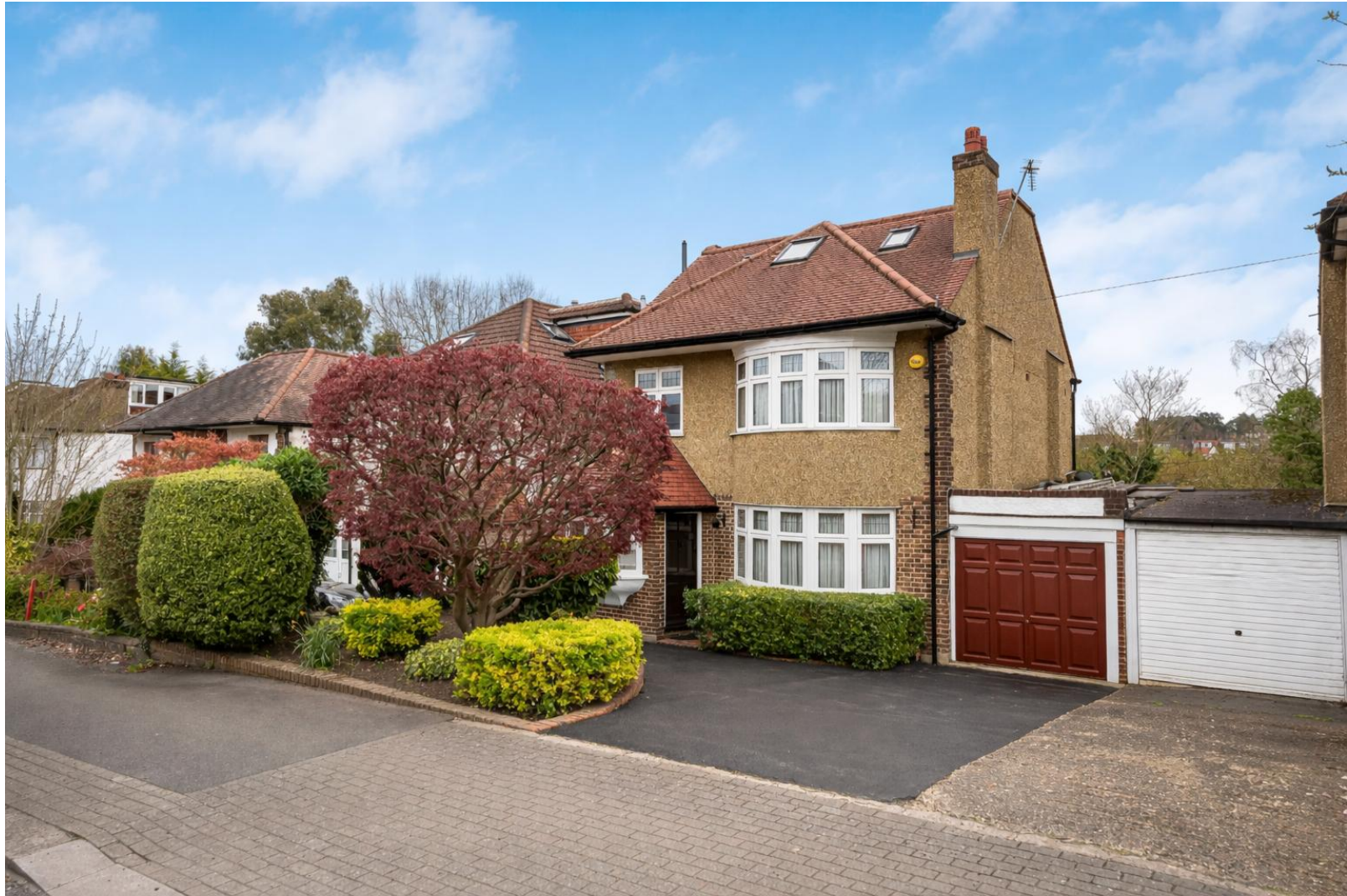
Longland Drive Totteridge, N20
