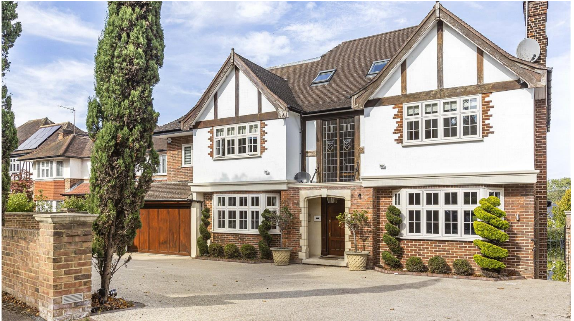
The Lodge, Lancaster Avenue, Hadley Wood, EN4 0ER
