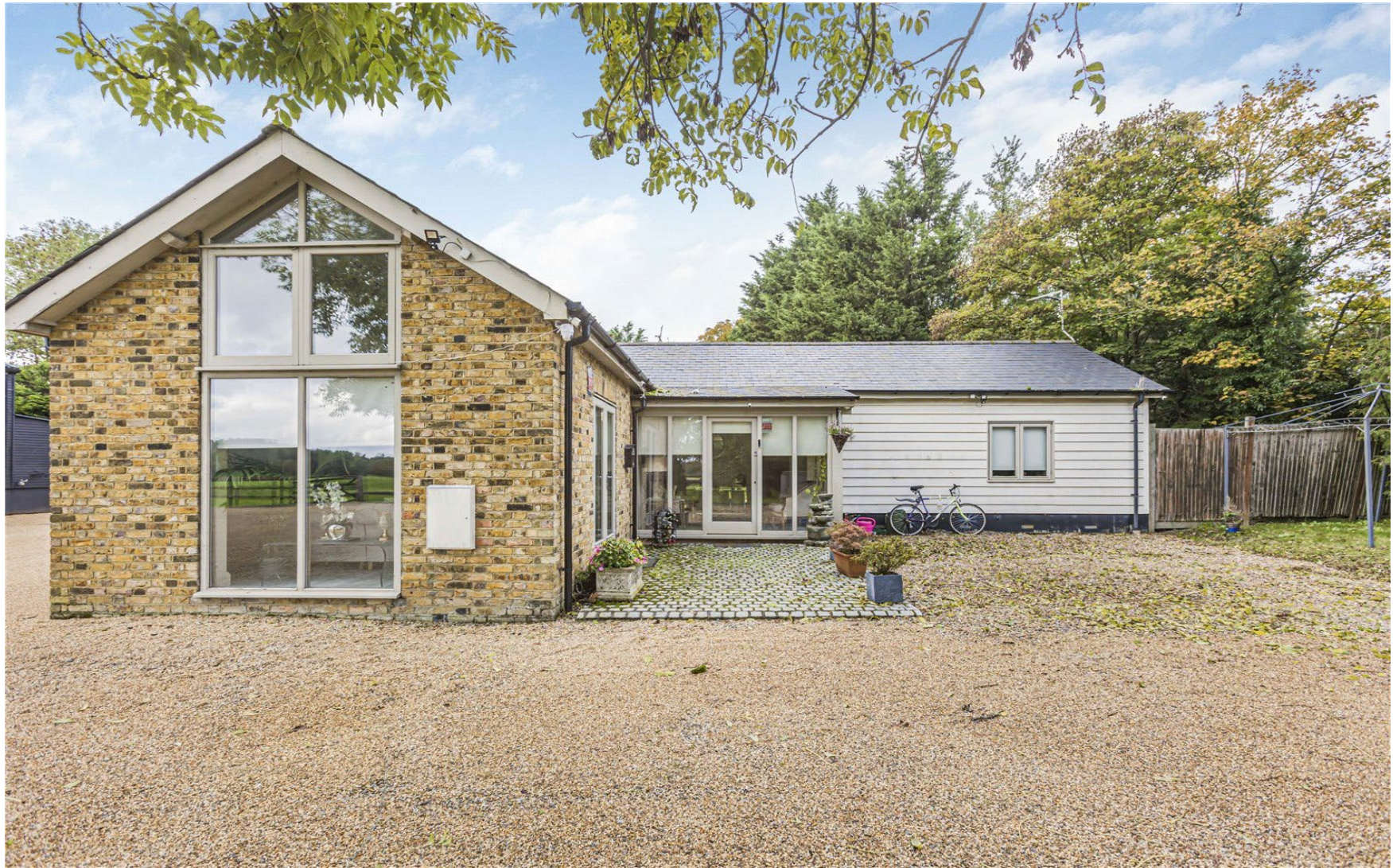
Lodge Farm Cottage Epping Green, Hertford, Hertfordshire.
