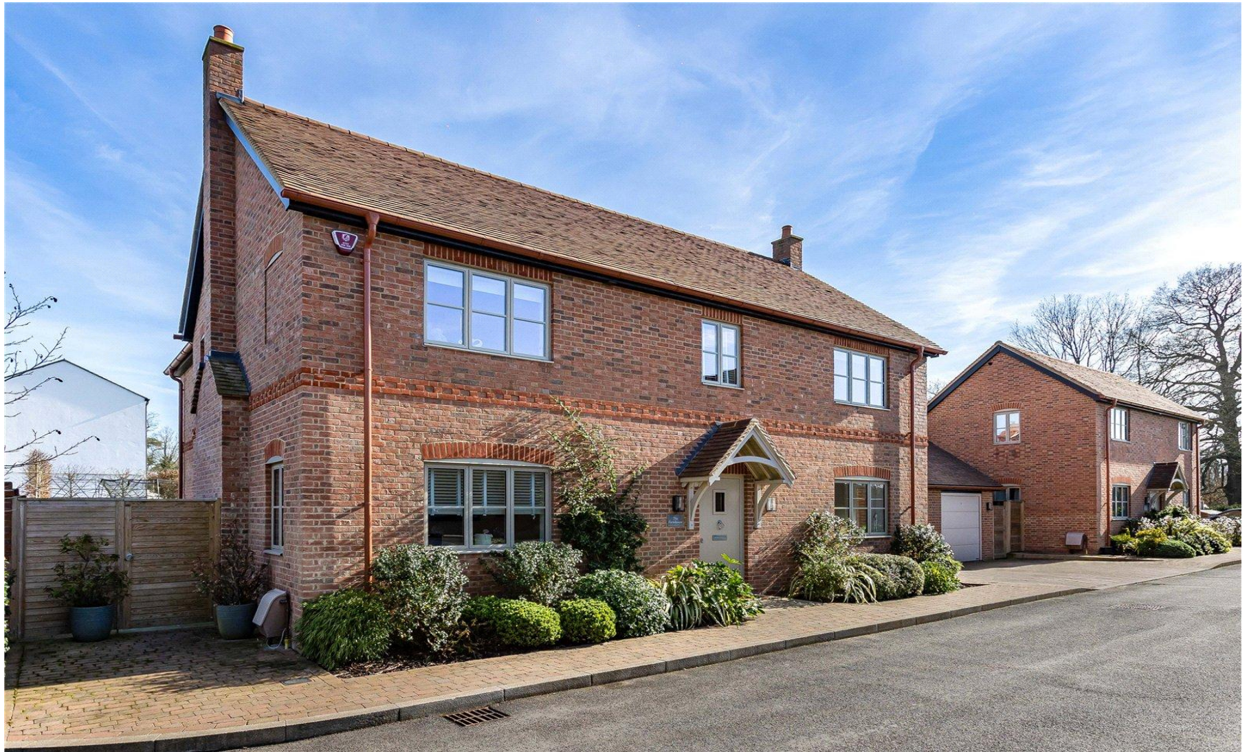
Northaw House Coopers Lane, EN6 4FG
