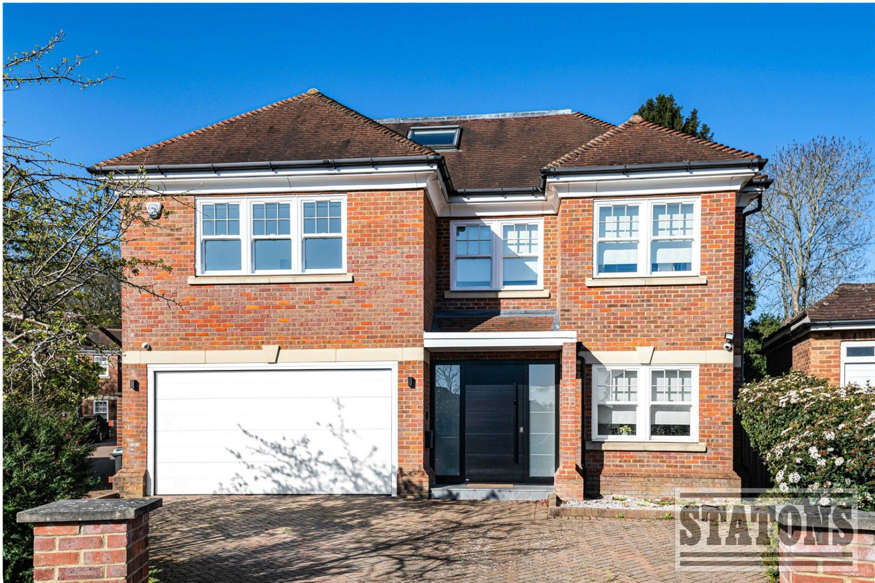
Parkgate Crescent Hadley Wood, EN4
