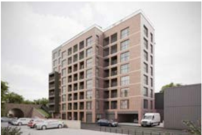
THE LINK APARTMENTS, BRENT CROSS
